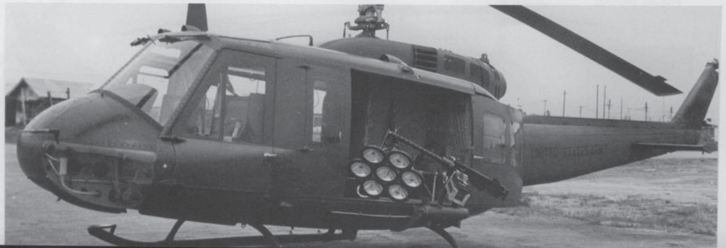
This UH-1D 'lightning bug' carries a hand fired .50 caliber machine gun for surpression fire. Although such heavy weapons were not normally fitted to the Huey, various experiments and field modifications were tried throughout the war to increase the helicopter's offensive firepower. (US Army)
